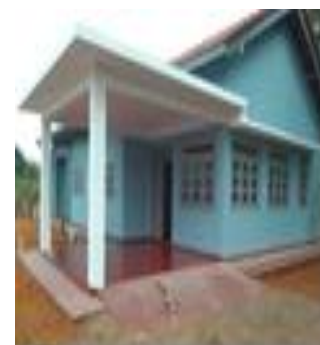
(ONUR) Construction of GHC Kokkuduwai centre Allocation: Rs.8.000M Expenditure: Rs. 6.400 M
