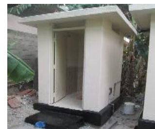
Development of sanitation facilities at Shantha Andruu Primary school, puttalam, Puttalam DS Allocations – Rs. 1100,000.00 Expenditure – Rs. 95,181.08
