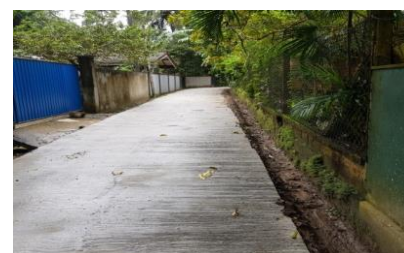
Concreted the Badalgewattha road at Meepe Allocations-Rs.460,350.00 Expenditure-Rs. 451,321.11
