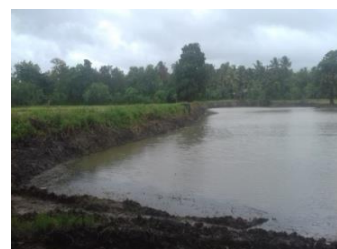
Renovation of upper tank at 485 Siyabhalawehera Gn Division, Ibbagamuwa DS division Allocations- Rs. 1,500,000.00 Expenditure – Rs. 1 500 000 00
