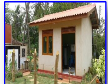
RO plant at Eppawala Sri sambodhi temple -Palugaswewa Allocations – Rs. 1.19M Expenditure 1.19M
