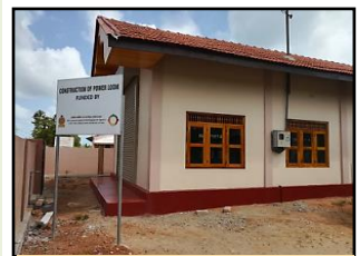
Power Loom Building Extension Work Tellippalai Allocation (Rs.) - 960,000.00 Expenditure (Rs.) -919,850.50
