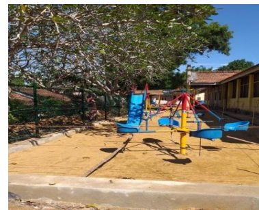
Construction of the playground at WelhengodaGunarathnaschool. Allocations-Rs.500,000.00 Expenditure-Rs.493,108.92
