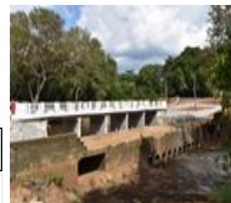
Reconstruction Paththukkan Bridge & Access Road
