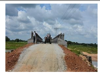
Project Name :- Construction of Bailey Bridge, Location :- Vellavalli Allocation :- 10.00 Mn Expenditure :- 9.90 Mn
