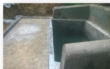
Construction of Mahawattahenagama well. Galigamuwa DS Allocations – Rs.300,000.00 Expenditure – Rs.395,000.00
