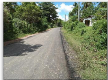
Laying the carpet road of near the Metigathwala temple Allocation-Rs. 24507685.70 Expenditure-Rs. 12030846.10
