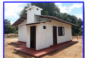
Construction 43 houses -597, Eppawala Allocations – Rs. 37.93M Expenditure – Rs. 37.93M
