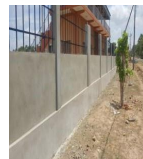
Construction of Boundary wall Kandawalai D.S division Allocations – Rs.1.60M Expenditure – Rs.1.57M
