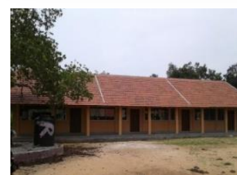
Construction of Class Room Building Manakandal GTMS Allocation-Rs.4.590M Expenditure-Rs.2.620M
