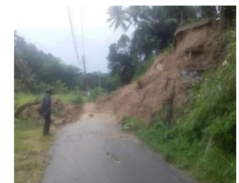
Facing emergency disasters
