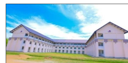
Three story building of Wilayaya Central College.
