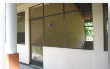
Modernize the polling centre of community building at minor fisheries villege –Nidahasgama East Allocation-Rs. 82400.00
