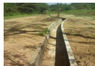
Renovation Kudahapollaanicut Allocation–Rs. 8.47M Expenditure – Rs. 6.80M
