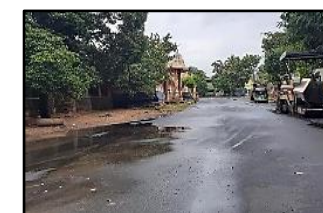
Construction of Inuvil Kandasamy Kovil Road Uduvil Allocations (Rs)- 24,607,421.03 Expenditure (Rs)-21,760,268.98
