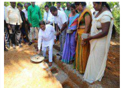
Laying foundation stone for Baddegama Nila sewana Building
